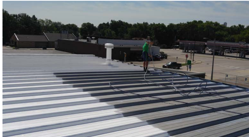
The Girard Middle School roof gets an application of Conklin roofing sealant.
